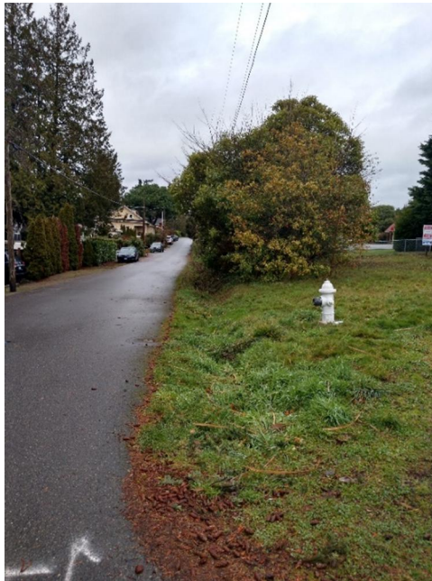
Photo S5 – Facing north on the east side of 62 nd Ave SE approximately 365 feet from Photo S4. Onsite runoff sheet flows in the southwest direction toward the ditch above and is conveyed south to be combined with the south basin downstream conveyance system.
