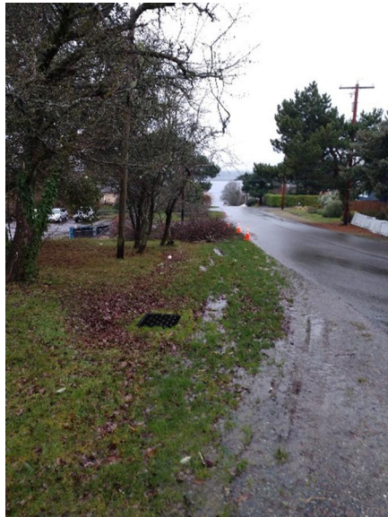
Photo N2 – Facing west along SE 28 th St approximately 170 feet west of Photo N1. Runoff continues to sheet flow northwest towards the conveyance system on the south side of the street.
