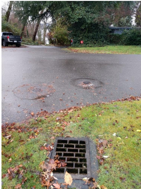
Photo S11 – Facing west along the north side of SE 30 th St approximately 130 feet west of Photo S10 at the northeast corner of the intersection of SE 30 th St and 60 th Ave SE. Runoff is conveyed west toward Lake Washington.
