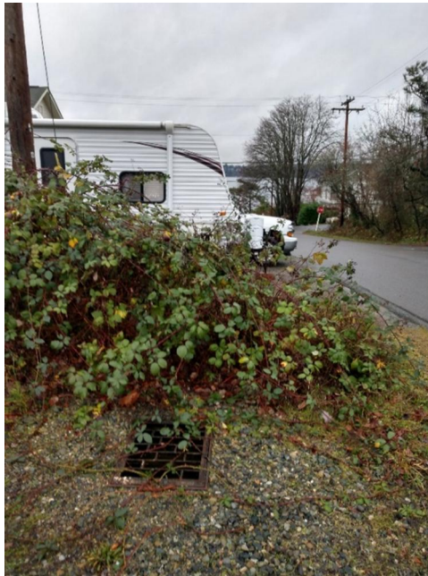
Photo N7 – Facing west along SE 28 th St approximately 90 feet west of Photo N6. Runoff is conveyed via this catch basin on the south side of the street toward Lake Washington.
