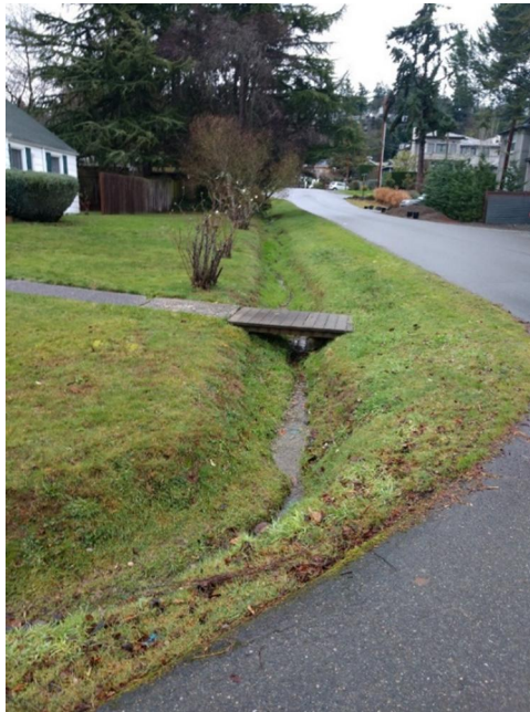
Photo S7 – Facing east along the north side of SE 30 th St approximately 210 feet west of Photo S6 at the northeast corner of the intersection of SE 30 th St and 61 st Ave SE. Runoff is conveyed west toward Lake Washington.
