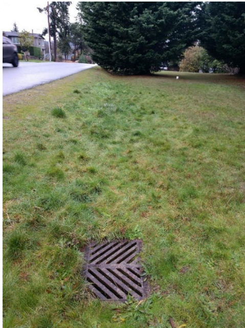
Photo S2 – Facing west along the north side of SE 30 th St approximately 55 feet west of Photo S1. Onsite runoff sheet flows in the southwestern direction to the catch basin above and is conveyed west toward Lake Washington.
