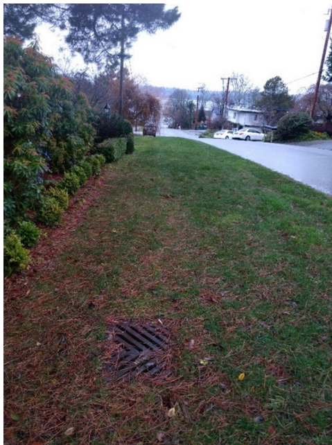
Photo N4 – Facing west along SE 28 th St approximately 130 feet west of Photo N3. Runoff is conveyed via this catch basin on the south side of the street toward Lake Washington.
