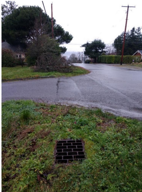
Photo N3 – Facing west along SE 28 th St approximately 145 feet west of Photo N2. This catch basin is located adjacent to the driveway into the back parking lot on the western portion of the property. Runoff continues to sheet flow northwest towards the conveyance system on the south side of the street.
