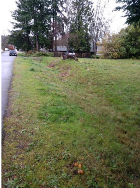
Photo S3 – Facing west along the north side of SE 30 th St approximately 35 feet west of Photo S2. Onsite runoff sheet flows in the southwestern direction to the ditch above and is conveyed west toward Lake Washington.
