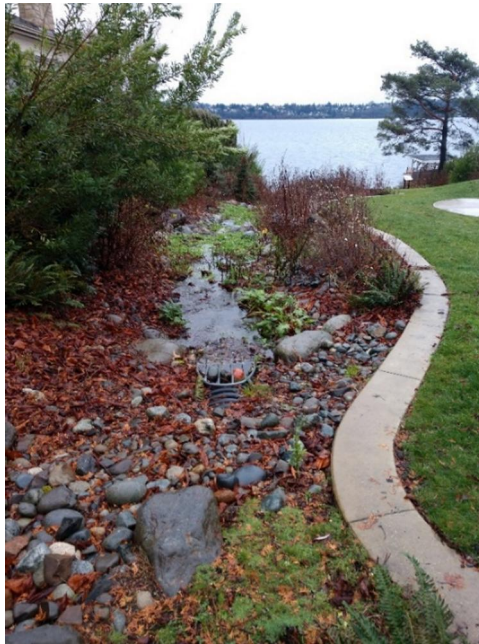
Photo N11 – Facing west in Calkins Landing. Runoff discharges via a pipe with a trash rack to a ditch upstream of the outfall to Lake Washington.
