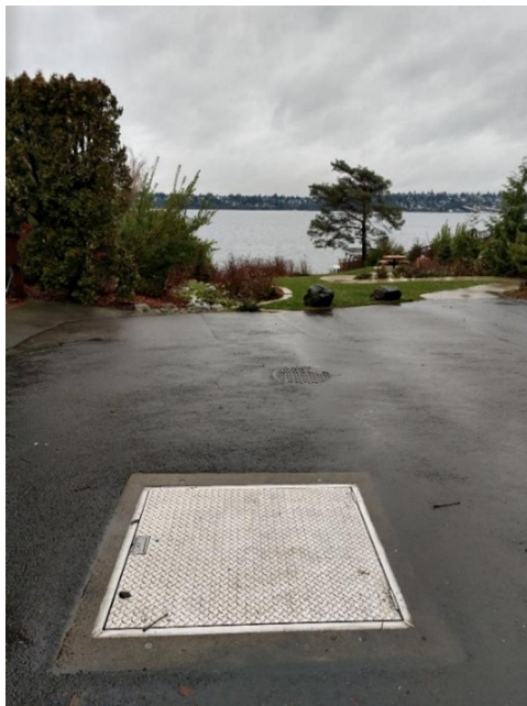
Photo N10 – Facing west in Calkins Landing approximately 95 feet west of Photo N9. Runoff is collected in the pre-settling vault pictured before being discharged into Lake Washington.
